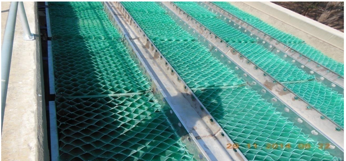
Figure 2: Lamella Tubes Installed in the Pre-settling Tanks at Walkers Ferry Treatment Plant
