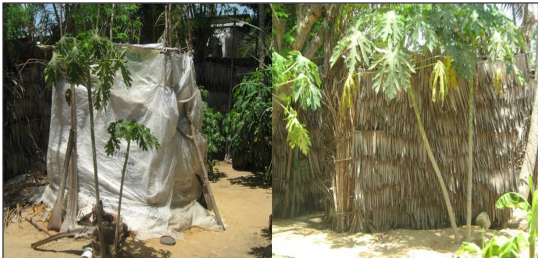
Plate 4.1-1: Bathroom constructed using plastic sheets and pit latrine constructed using Palm thatches
