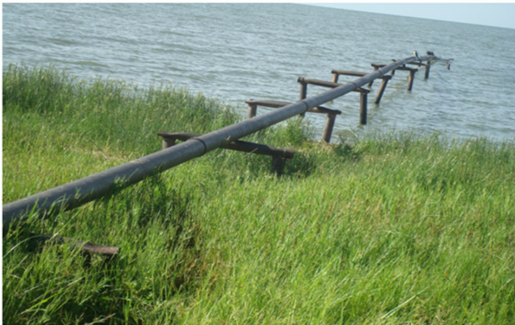
Plate 4-2: Long suction pipe due to lowering of Lake Victoria water level-Isanju village
