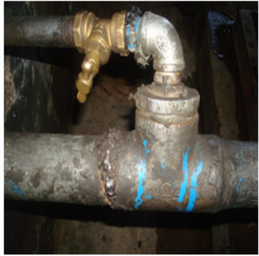
Plate 4-3 and 4-4: Forged spare parts and the threaded Joint is welded at Kibara Scheme
