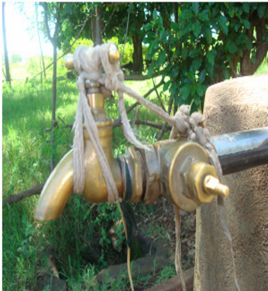
Plate 4-5: Improper O&M of DP at Bulendabufwe Gravity scheme
