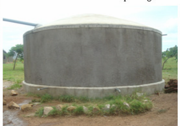
RWH tank without bib cock and plug-Sazira Sec
