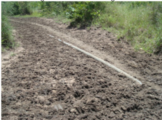
Uncovered PVC gravity flow main on cow trail Bulendabufwe gravity scheme
