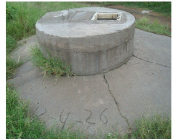
Vandalised shallow well hand Pump-Kung'ombe
