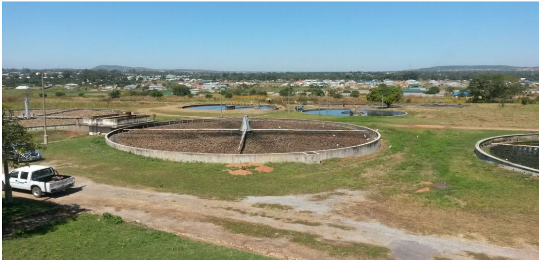
Figure 4. 1: Kanini Sewerage Treatment Plant (Capacity of 11,000 m 3 /day)
