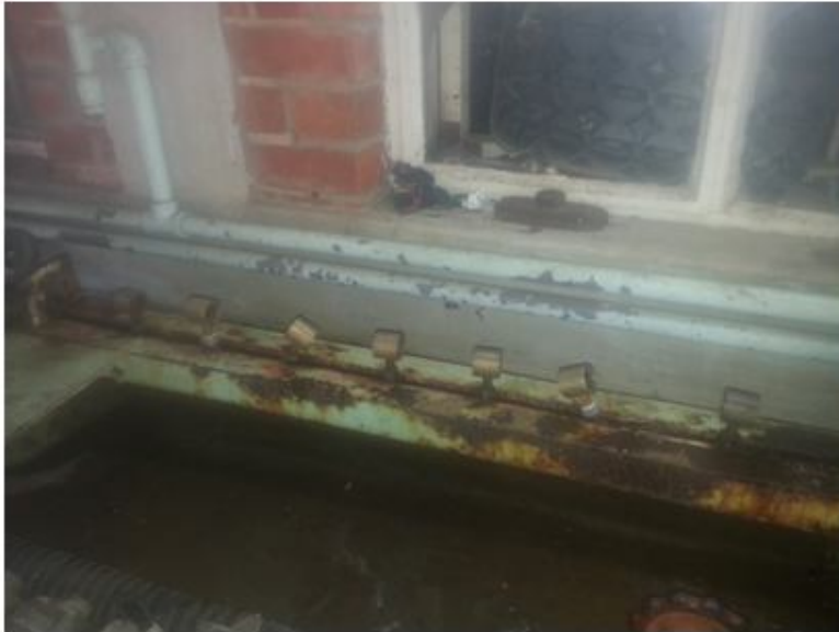
Meter testing Bench- before testing
